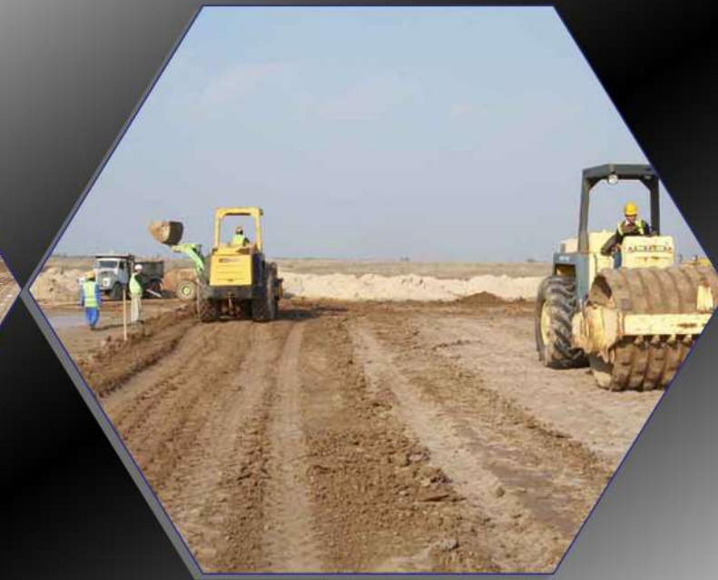
Burying and leveling of wells and road construction
